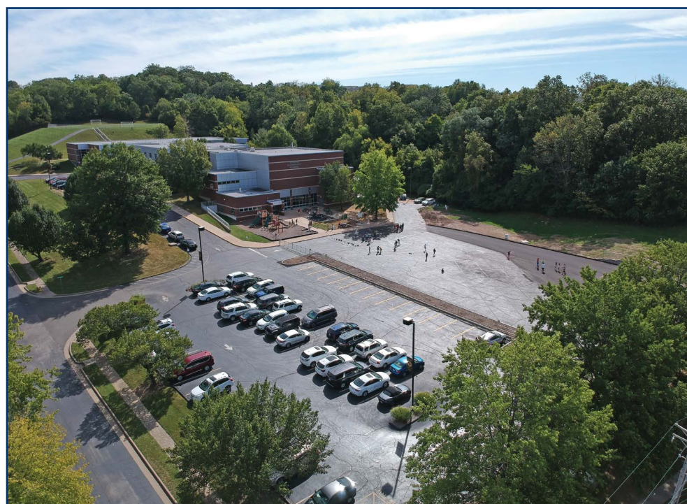
A concrete barrier now separates the Rogers Elementary School parking lot and playground.
