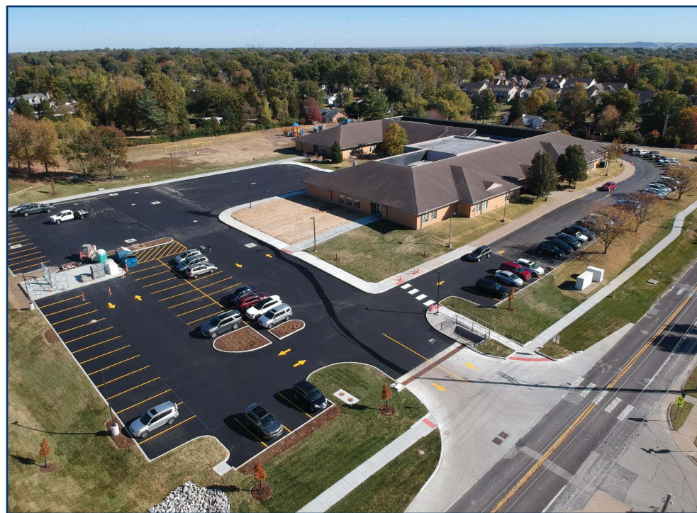
Oakville Elementary School's expanded parking lot was completed last month.
