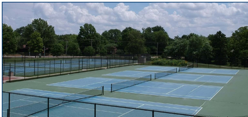
Crews repaired cracks in the tennis courts at Bernard Middle School this summer. The courts were also repainted and new nets were added.
